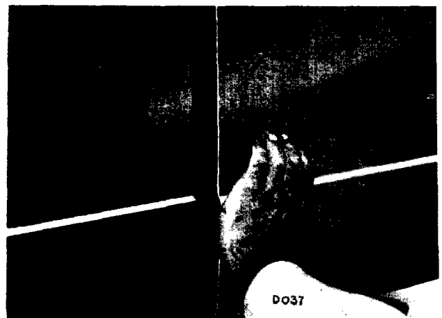
Fig. 60. Inserting wedges to increase gap
