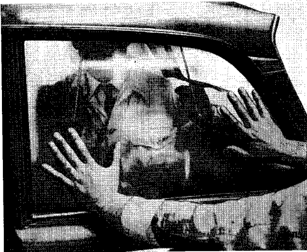
Fig. 86. Fitting quarter light
