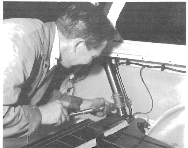
Fig. 105. Removing fuel tank (Estate car and Van)
