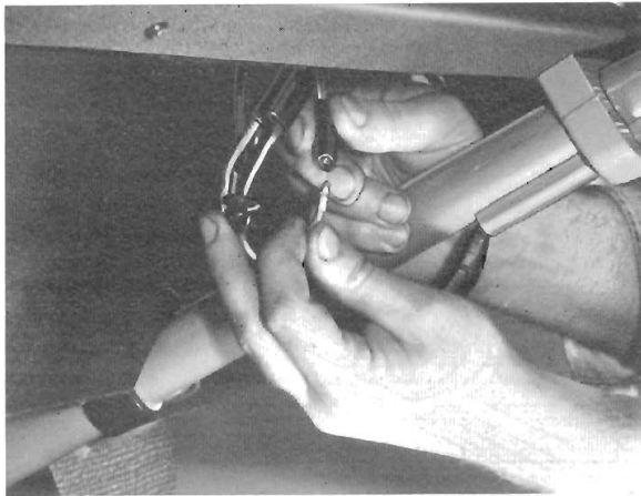
Fig. 30. Reconnecting cables at snap connectors
